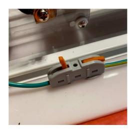
1. Once you have removed the left side panel, unclip the cable from the cable connector at the front of the unit. Lift the orange lever tag (as shown above). The cable will slide out freely.
